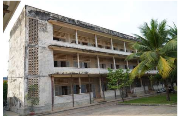
View of Building C, Tuol Sleng Genocide Museum (TSGM)
